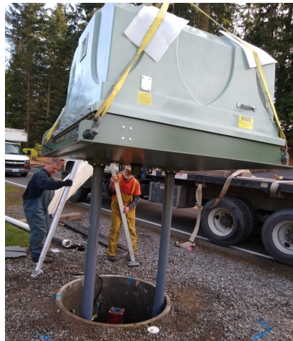
Installation of new Taylor Lift Station
